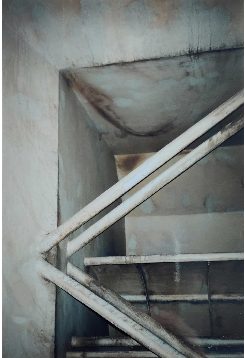
Above the top of the Elbow is shown where there are visible results after turbulence at the outer radius of the Elbow, which is not common.
