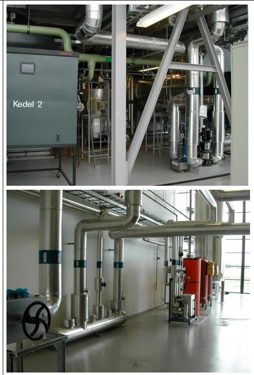
Pictures from a Steam Boiler Plant for a Pharmaceutical Factory (Denmark). There were 3 off heating system. Circulation was handled with one Skid Mounted Unit.
