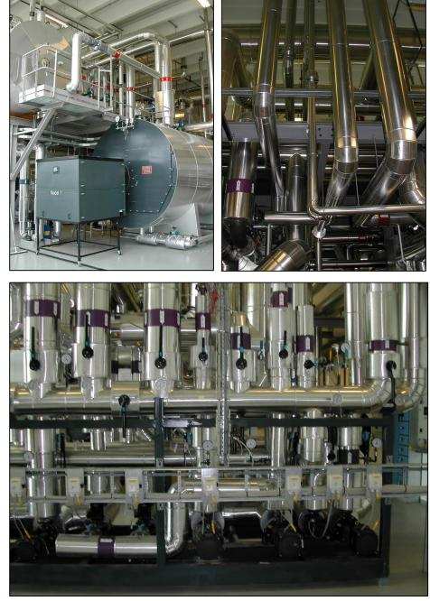
Pictures from a Steam Boiler Plant for a Pharmaceutical Factory (Denmark). Production of 2 times 10 barg Steam @ 8 barg for distribution in plant.
