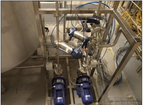
Pictures from a Neutralization Plant in a Pharmaceutical Factory in Denmark. Designed for batch operation receiving both raw water and purified water. Contract performed as EPC.
