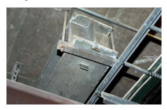
The old concrete structure could not take the same load as specified for the removable platforms sections. To reinforce the concrete structure a frame of steel section was applied around the holes transferring the loads away from the edge of the concrete floor.
