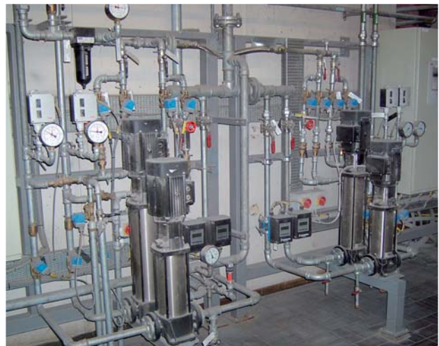
Two units on one skid supporting 2 boilers.
