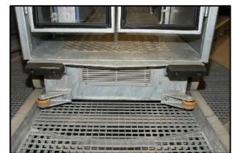
Pictures from the Harbor Tunnel in Copenhagen.
