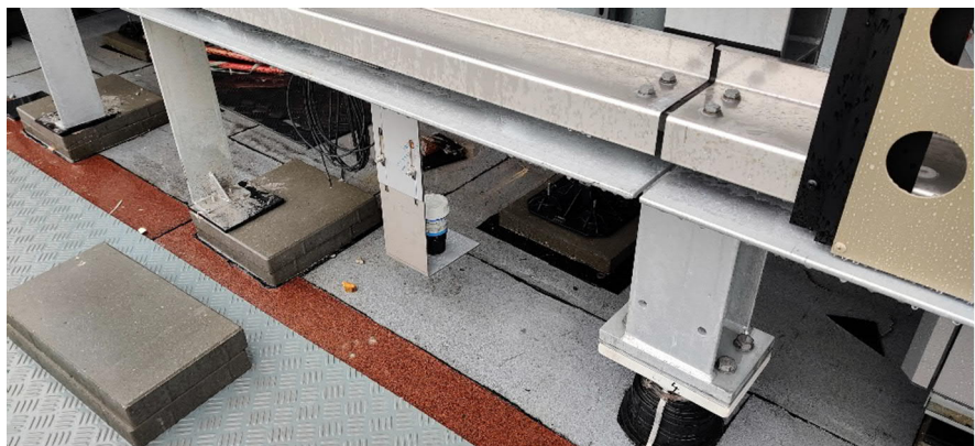
Support Points and integrated fixture for Level Switch
