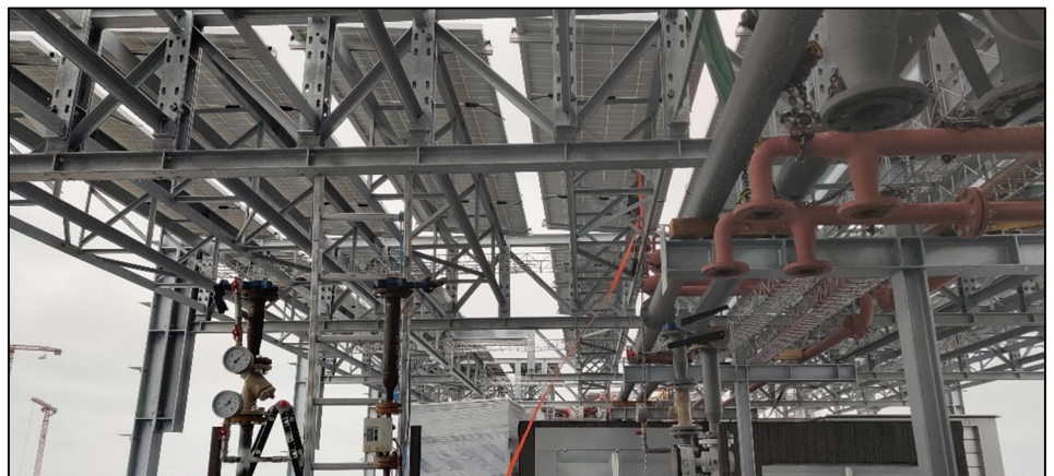
Top Picture shows a snap of a 3D Detail Drawing of a Steel Structure supporting 2 off Silos and Prepared for mounting Cover Plates for Machinery Room beneath. Below steel structure for a Roof House for Technical Installations with a cassette system for erection Solar Panels easily.
