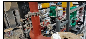
Pictures from DFDS HQ Built by NCC.
