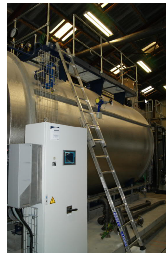
Top Pictures from a Pharmaceutical Plant with Flue Gas Condensation for Supplementary Heating Production. Bottom Picture from an API-factory with 2 step Flue Gas Cooling for both Cooling Production and Supplementary Heating Production.
