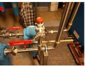
Pictures from Compressed Air Installation at a Pharmaceutical Factory (DK). For this project, the Consulting Engineer had Specified a Pipe Series without Tees etc. and therefor Special Nozzles had to be manufactured.
