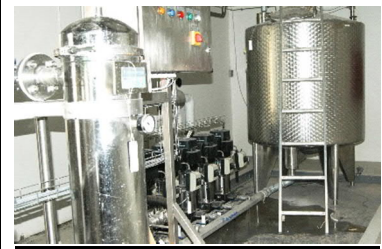
Examples from prefabrication of Water Piping:
