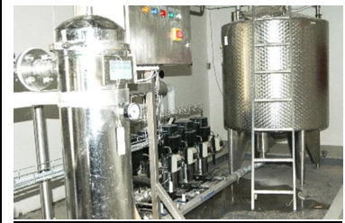
Examples from prefabrication of Water Piping:
