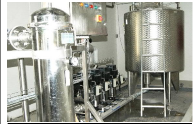
Examples from prefabrication of Water Piping:
