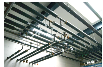
Pictures of various Pipe Insulation and insulation Specification H03, which covers e.g., indoor heating installation.
